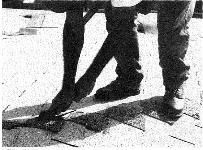
Figure 4-20 Trimming the hip
