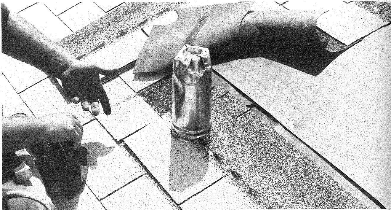
Figure 4-73 Embed the overlying shingle in roofing cement
