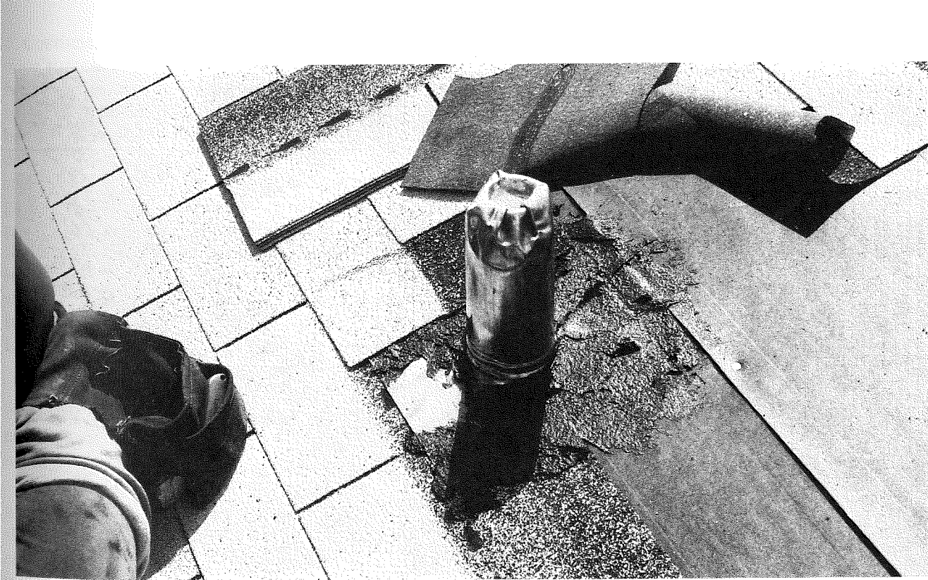
Figure 4-72 Embed the flange in roofing cement
