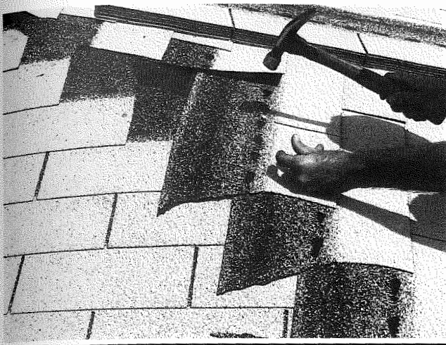
Figure 4-19 Lapping shingles over a hip
