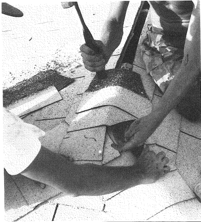
Figure 4-45 Cut the ridge unit and nail down one flap
