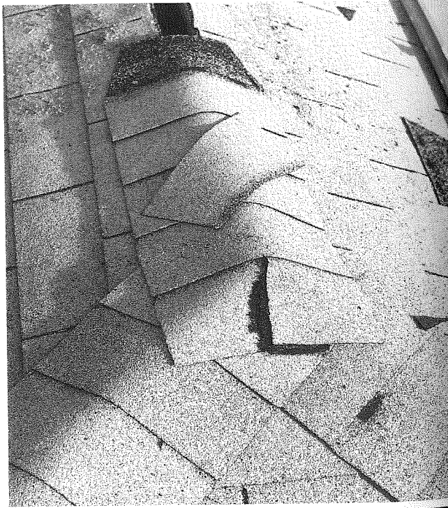
Figure 4-46 Seal the hip-ridge junction
